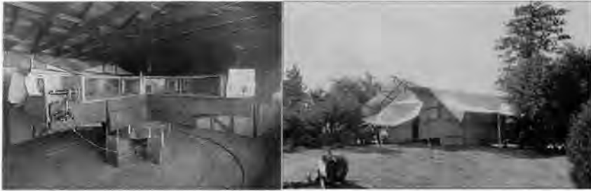
Figure 4. Left: Miller's fully-insulated interferometer as it was finally employed at Mt. Wilson, circa 1925, fitted with 2.5 cm insulating cork panels covering the metal support structure, and glass and light paper coverings along the light-beam path (paper removed for the photograph). These steps eliminated any significant influences of ambient temperature differences upon the apparatus and the air within the light-beam path, but still allowed the movement of ether-drift. Right: Miller's interferometer house on Mt. Wilson. With canvas-covered windows all around, insulating wood fibre walls, and fitted with a tent.
