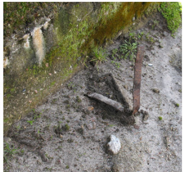
Fig. 12: Mounting bolts for one of the legs of the mast (left), and embedded ground
