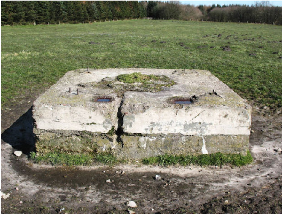
Fig. 11: Concrete foundation of the monitoring-antenna mast (right-hand photo: the mast was partly re-used later)
