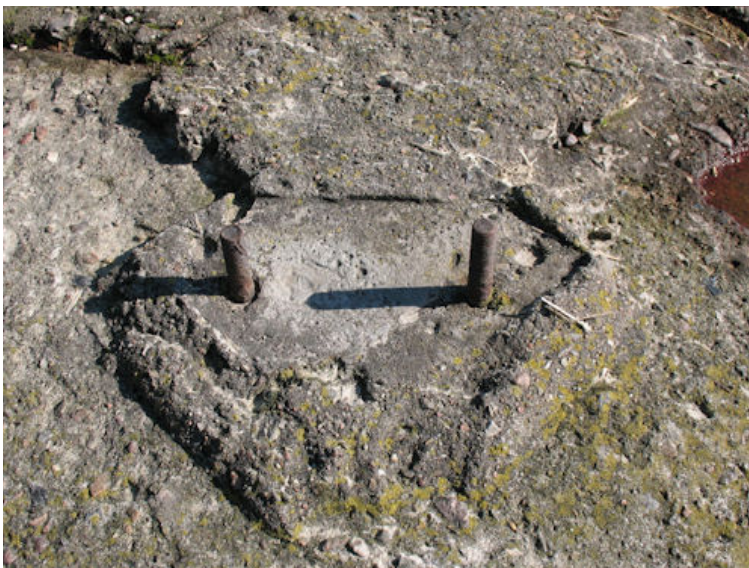
Fig. 12: Mounting bolts for one of the legs of the mast (left), and embedded ground
