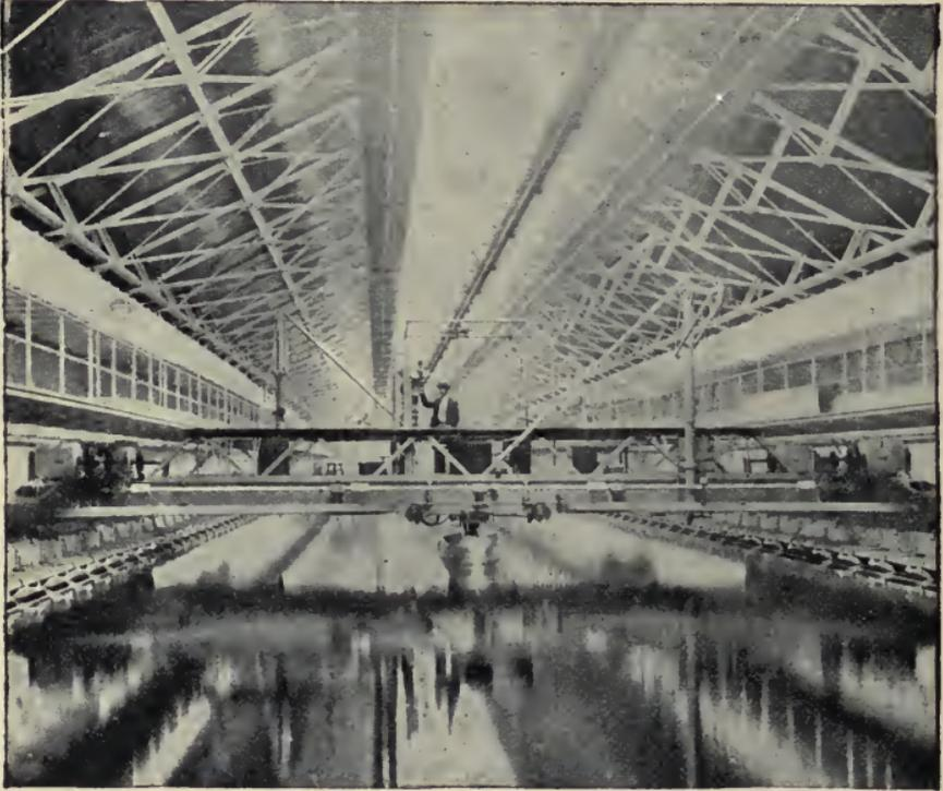
FIG. 40.—An experimental tank for testing ship models (Washington).\*
