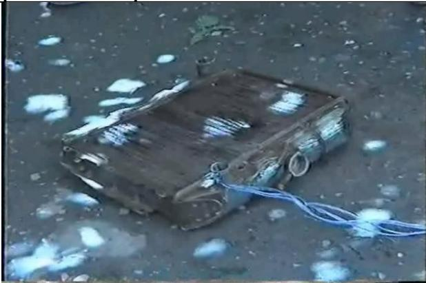
Figure 5. Grounding radiator
