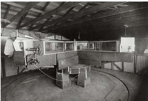
FIG. 8. **Miller's fully-insulated interferometer** as it was finally employed at Mt. Wilson, c.1925, fitted with 1" insulating cork panels covering the metal support structure, and glass and light paper coverings along the light-beam path (paper removed for the photograph). These steps eliminated any significant influences of ambient temperature differences upon the apparatus and the air within the light-beam path, but still allowed the movement of ether-drift.
