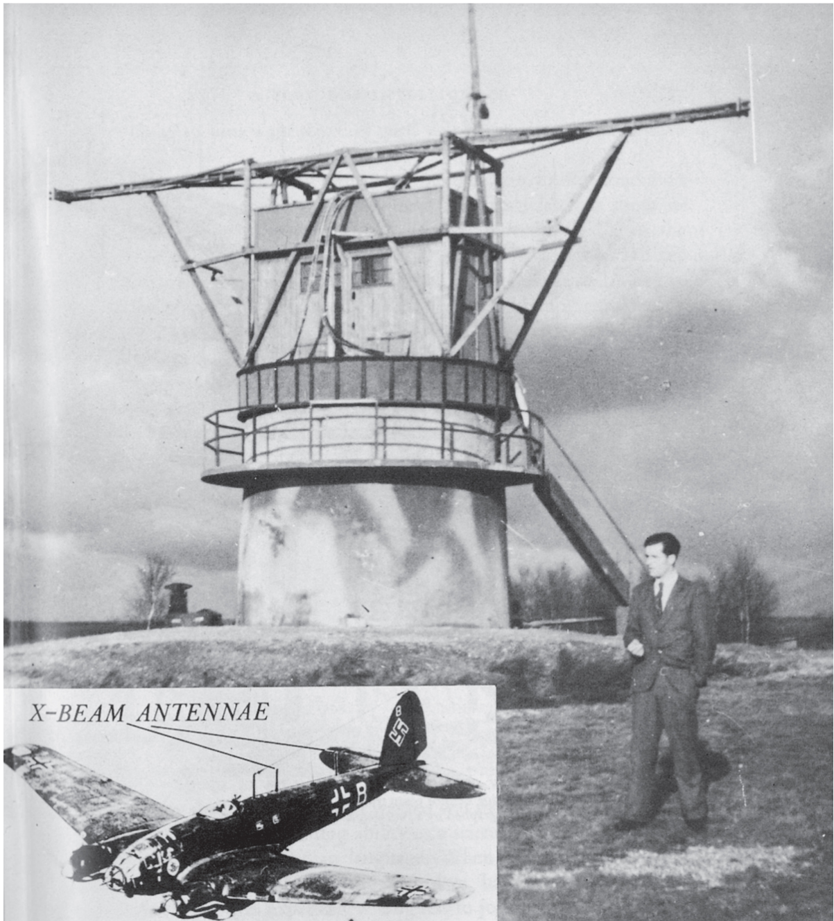
7. A Wotan I or X-Beam transmitter. Inset: A Heinkel III with receiving antennae for X-Beams (Photographs courtesy of F. Trenkle).
