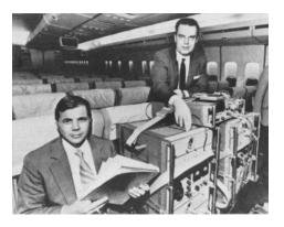
The experiment consisted in using two high precision Caesium atomic clocks, synchronised with a US reference ground station (USNO) for flying them on commercial aircrafts for two separated closed flight trips, one eastward, and one westward. After returning to USNO the clock times were compared with the reference time and the time shifts recorded. The observations were compared with the predicted values calculated applying the general relativity formula and a close matching was found.
