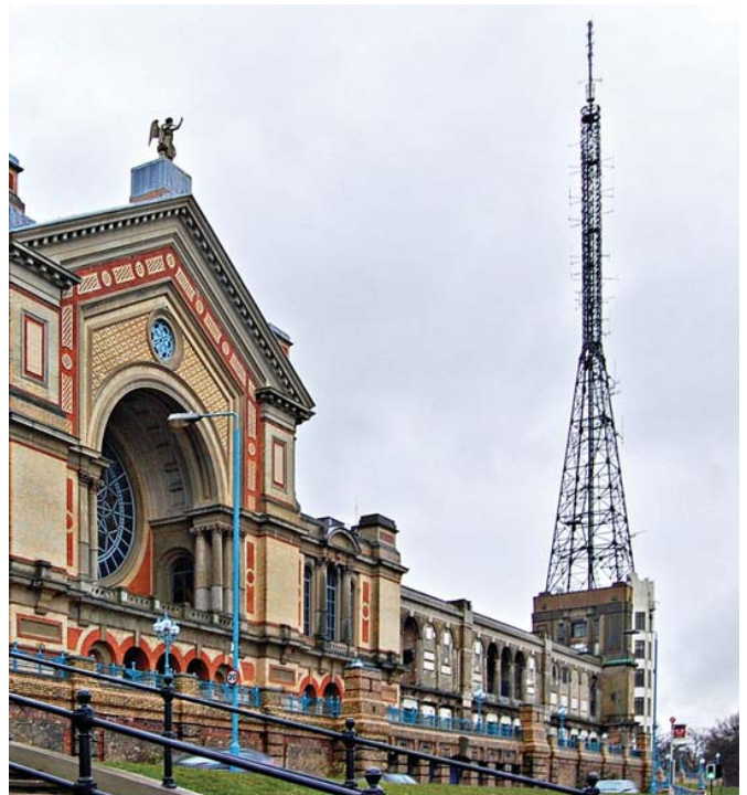
The Alexandra Palace TV transmitter was used to disrupt Y-Gerät on 42.5MHz. (Photo based on Duncan Harris/CC-BY-2.0).
