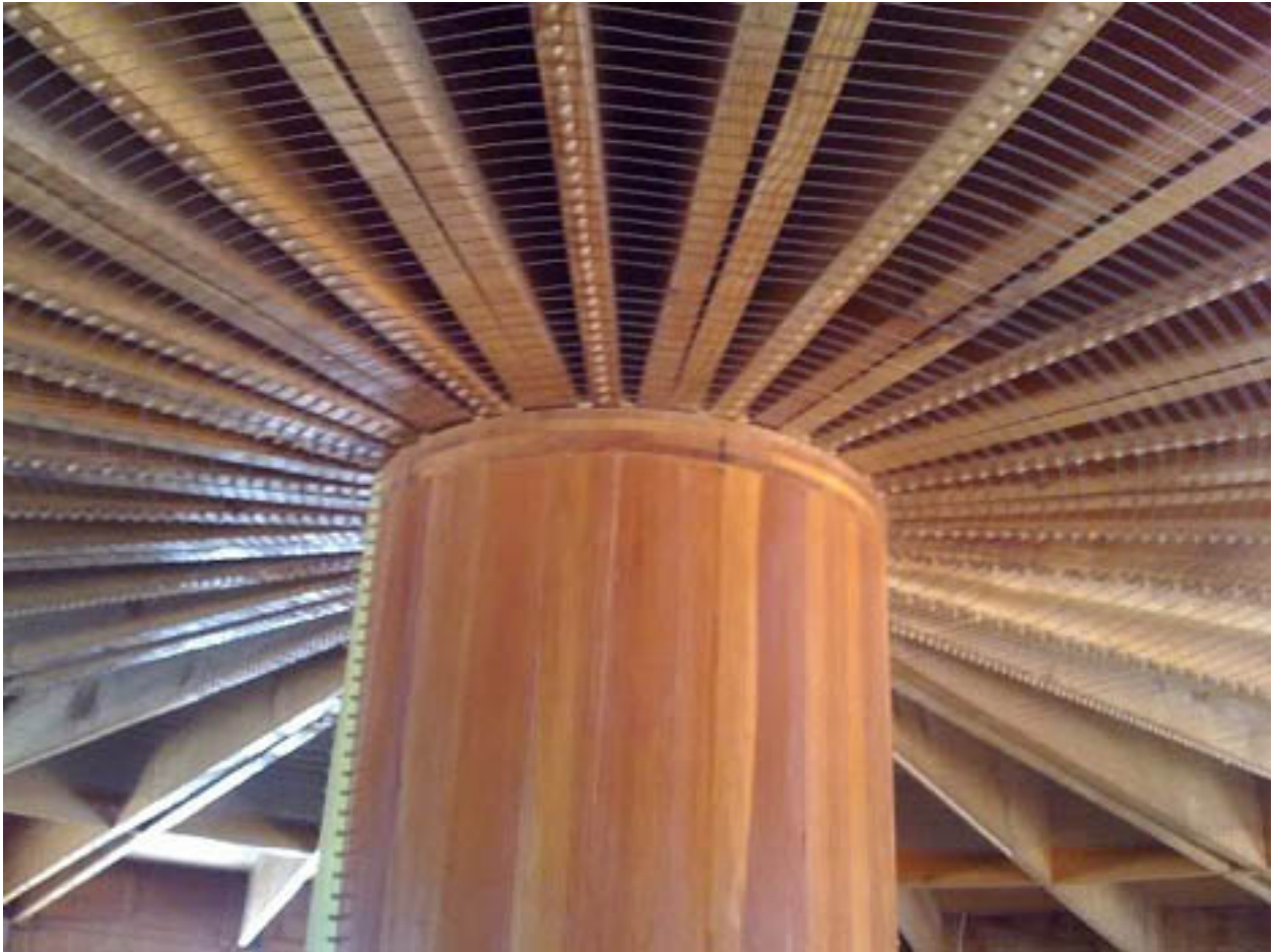
INTEGRATRON – CEILING TRANSFORMER WINDINGS & CENTRAL COLUMN Figure 34
