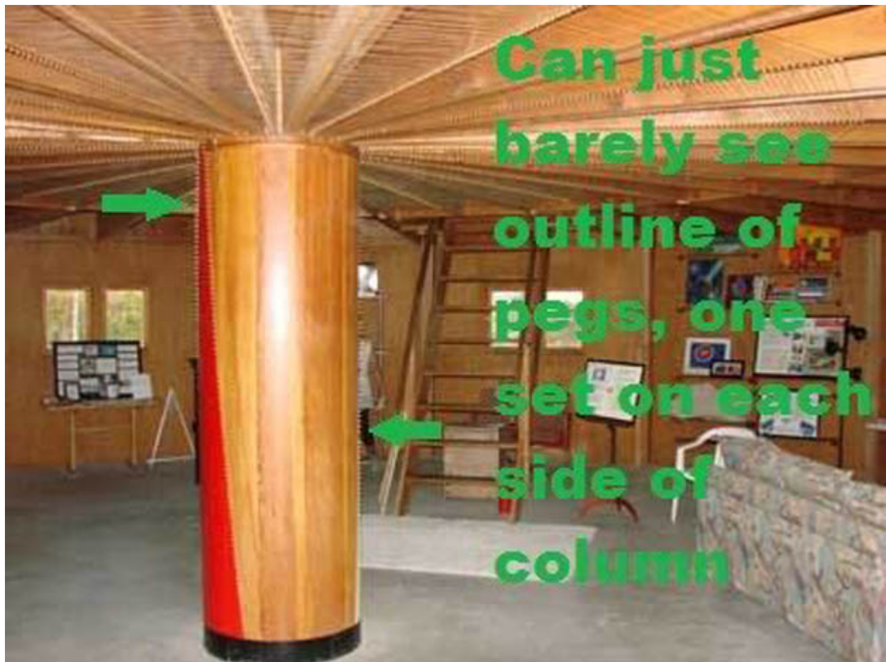
INTEGRATRON – TRANSFORMER DETAIL CENTRAL COLUMN CONDENSER (RED)
