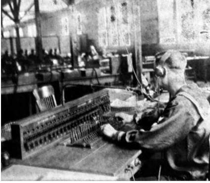
Fig. 21. Operating table telephone switchboard for instruction at Harvard Radio School. ( Oscillator , Jan. 11, 1919, p. 15)
