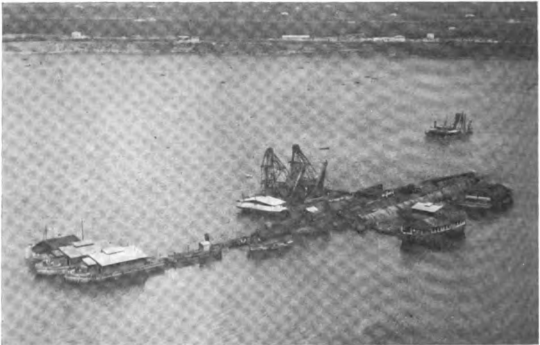
GENERAL VIEW OF WORK PRIOR TO DOCKING.
