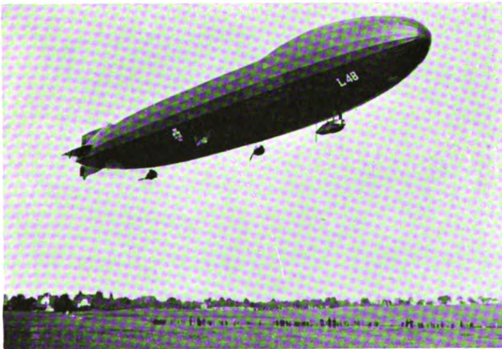
FIG. 4.—1916 Type Zeppelin ( L-48 ). One of this Class was Forced to Land in France and Became the Source of much Valuable Information for the Allies. Lower Half of Ship is Dark Colored for Night Operations.
