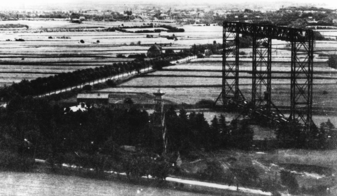
The huge Knickebein beam-transmitter at Stollberg in Schleswig-Holstein. The aerial array was about 100 feet high, and was supported by railway bogies which ran on a circular track 315 feet in diameter to align the beam on the target.
