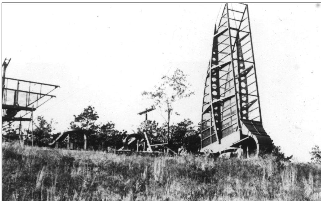
Above: The 'Tuba' equipment, designed and built at the Radio Research Laboratory at Harvard, was the largest and most powerful jamming system produced during World War II. The man standing at the base of the aerial gives scale to the special directional array developed for the jammer. 'Tuba' became operational too late to have any effect, however.
