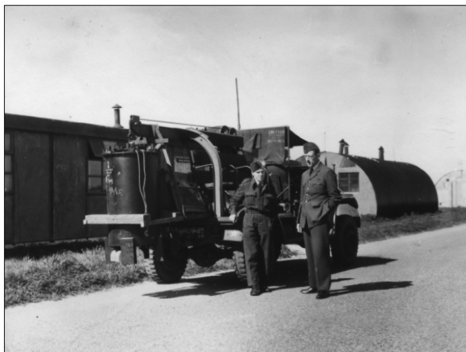
Above right: The 600-pound cylinder of the 'Jostle' high-powered VHF communications jammer, mounted on the rear of its special transporting truck. This jammer was fitted to the jamming escort Liberators and Flying Fortresses of No. 100 Group.
