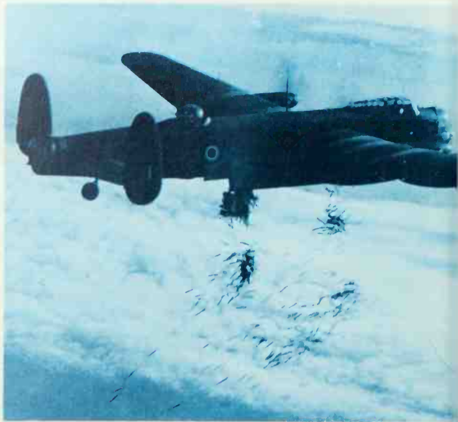
Above: Incendiaries cascade from one of the highly secret B.I.s of No 101 Sqn, from Ludford Magna, with Airborne Cigar electronic jamming equipment (note the two tall dorsal masts).
