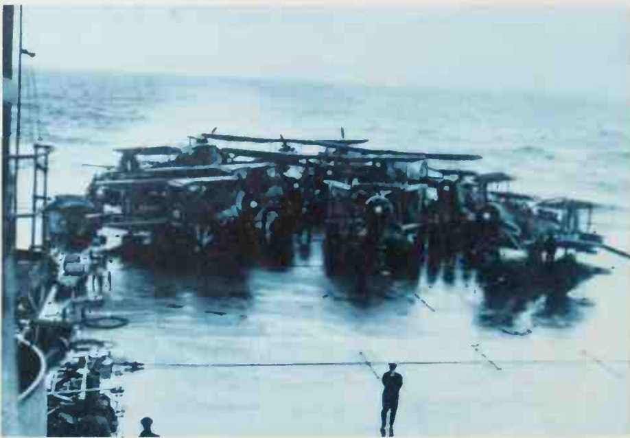
Below: Probably taken in early 1942, this scene shows "Stringbags" huddled on the constricted deck of an escort carrier.
