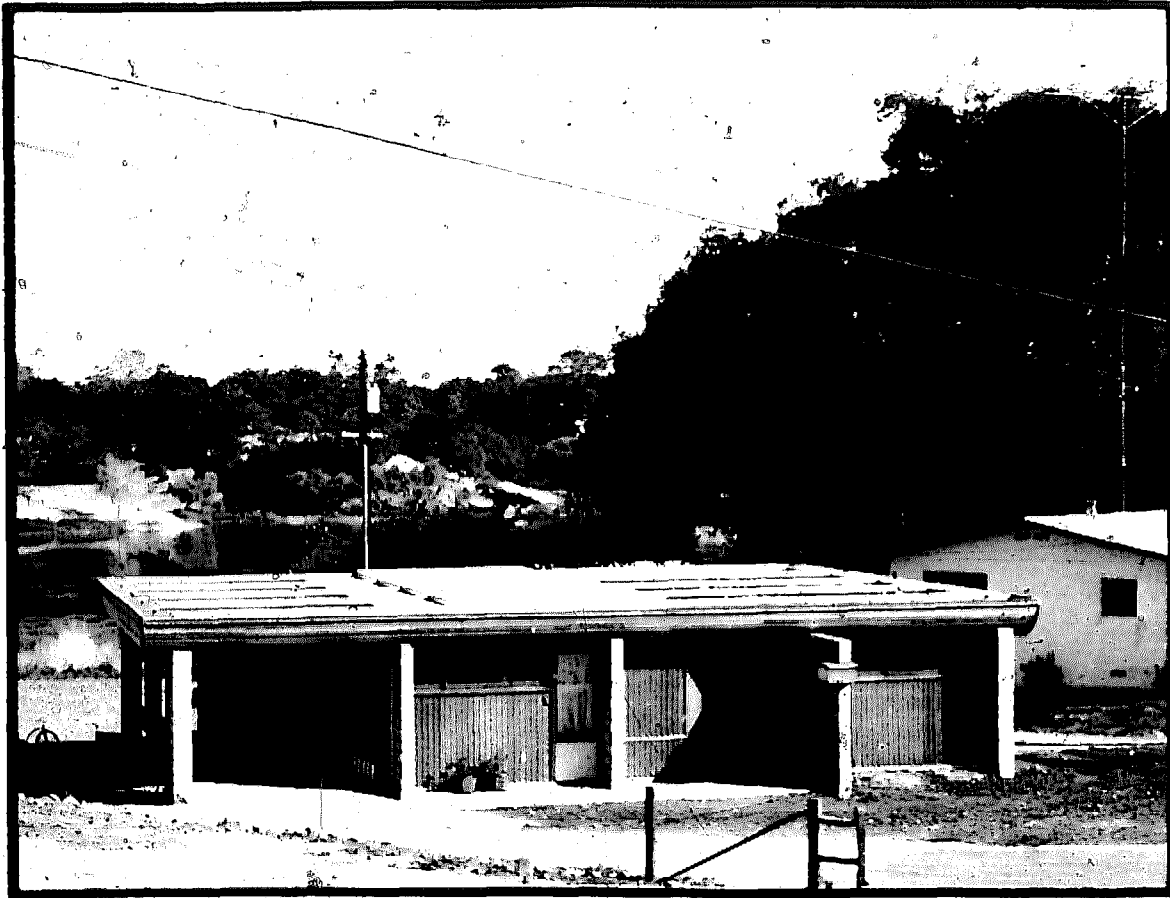
Photo III-9: Atascadero residence—first residential prototype incorporating a roof pond system.
