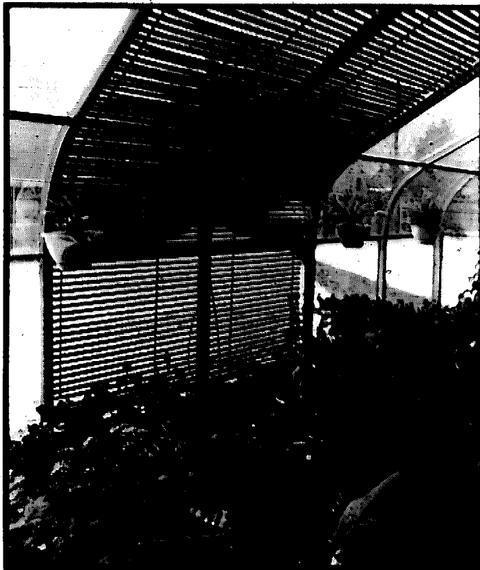
Photo IV-20e: Louvered shading device.
