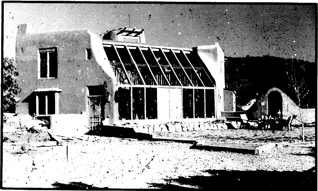
Photo IV-15c: Building surrounds the greenhouse to reduce the exposed exterior surface area.
