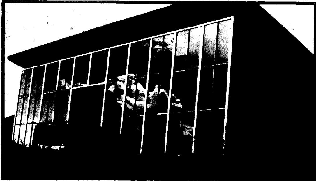
Photo III-5: The first Trombe house (above); attached housing units with thermal storage walls, Odeillo, France (below).
