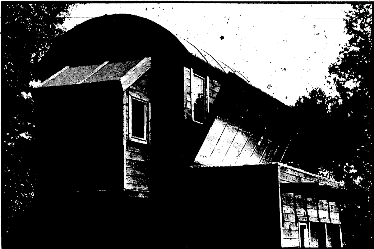
Photo IV-17b: Winter daytime position of reflector/insulating panel.
