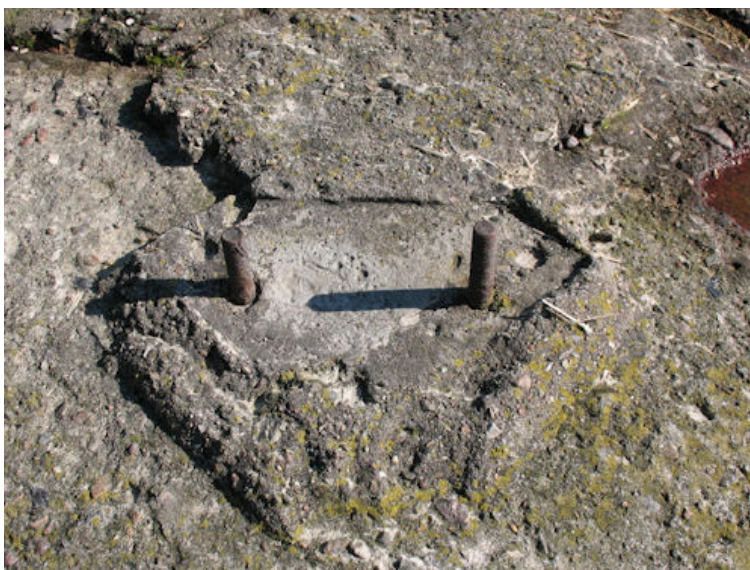
Fig. 12: Mounting bolts for one of the legs of the mast (left), and embedded ground
