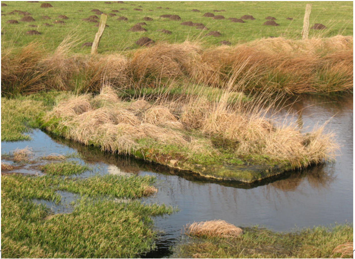
Fig. 9: The rectangular concrete foundation of the power generator is still still there (source: ©2008 R. Grzywatz, used with permission)
