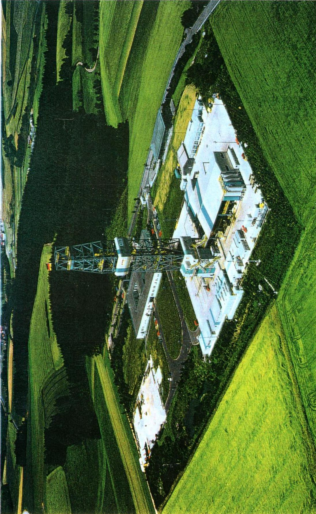
**Plate 1.** Aerial view of the KTB drill site with the drill rig of the superdeep hole in the foreground. The site of the pilot hole is to the left, 200 m from the drill rig. The field laboratory occupies the main building in the background.
