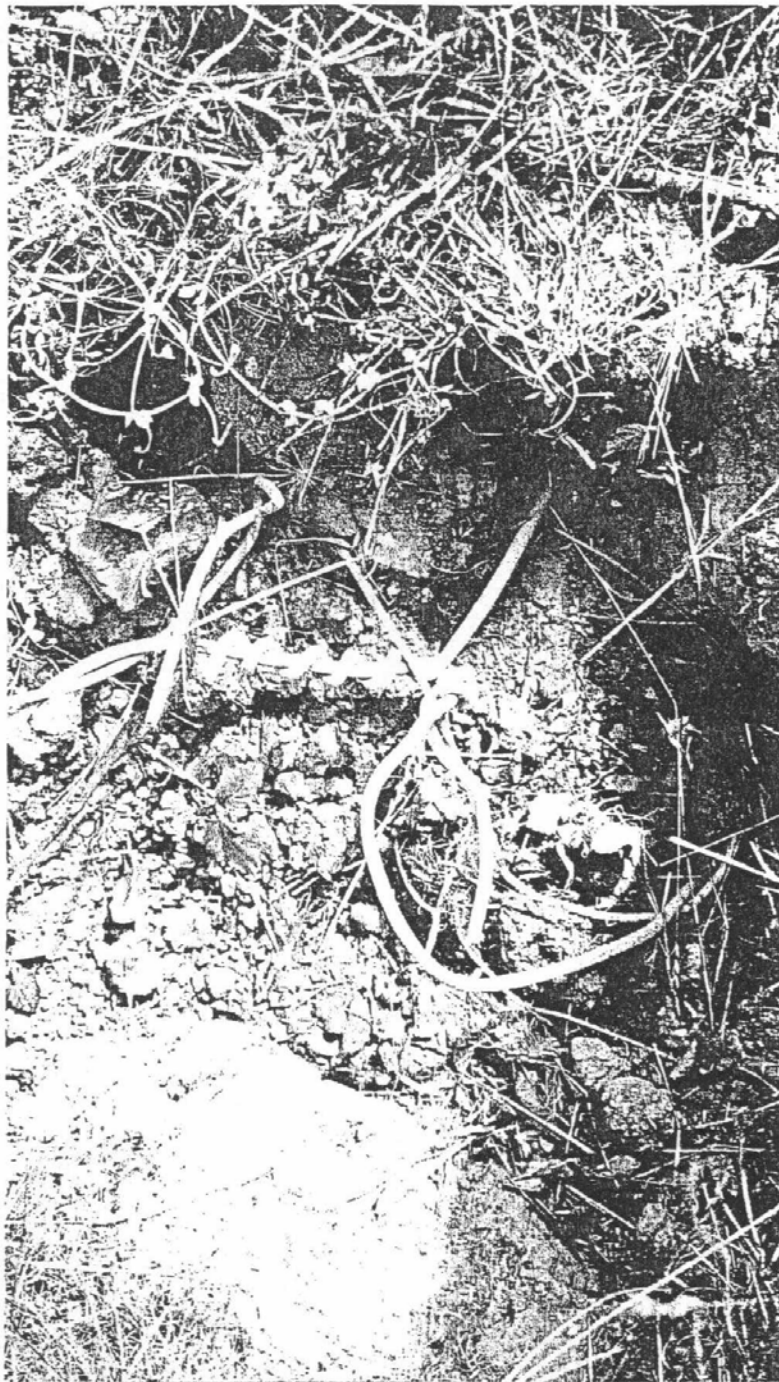
PTB/ Fig. 32: #4 ground wires
