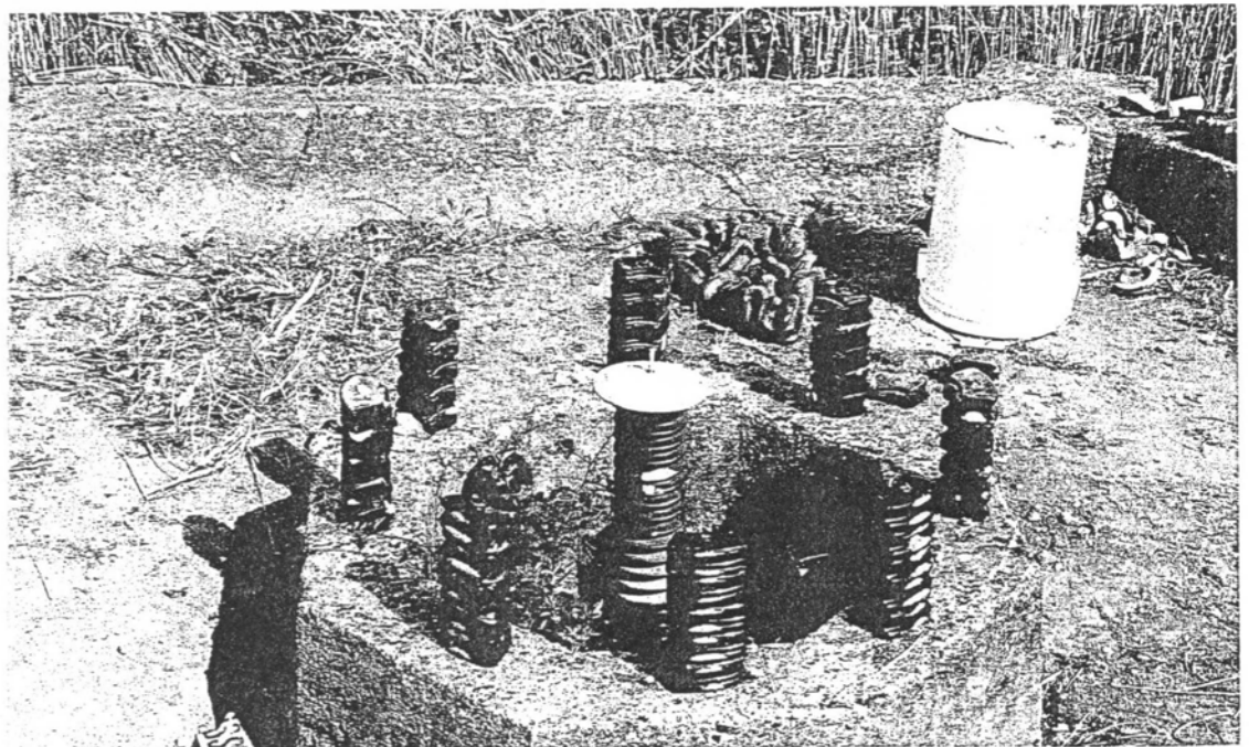
PTB/fig. 37 D : unknown shack Foundation Series coil insulators stacked as in use
