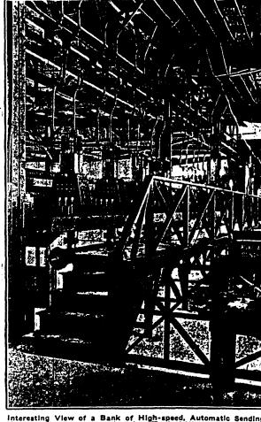
Interesting View of a Bank of High-speed, Automatic Sending Keys and Bus-bar Connections in a Typical High-power Narconi Radio Station.
