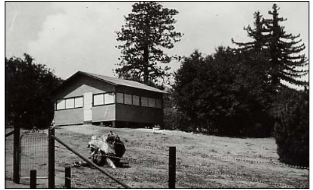
FIG. 9. Miller's interferometer house on Mt. Wilson. Top photo: with canvas-covered windows all around, and insulating "beaver-board" walls (wood fiber composite). Bottom photo: the same house fitted with a tent cover over the roof and walls to further stabilize temperatures.
