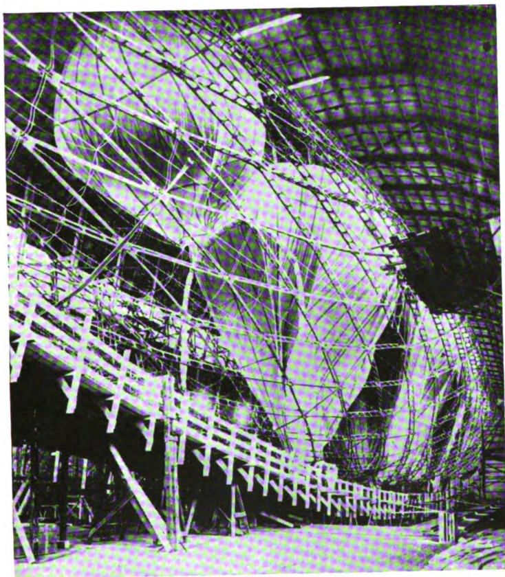
FIG. 1.—Skeleton of SL-1 . Gasbags Partially Inflated. Note Spiral Framework.
