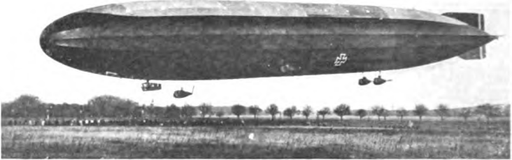
FIG. 8.—Late (1917) Type Schutte-Lanz Ship. 1,978,000 cubic feet Capacity.
