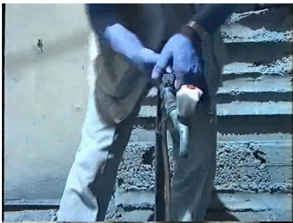
Figure 6. Using a water pipe as a ground connection
