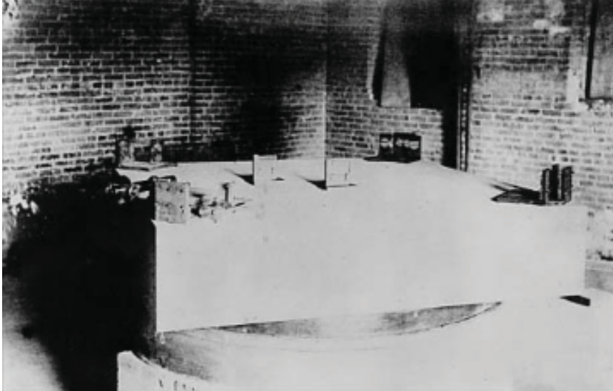
Figure 4. The original Michelson-Morley interferometer with an approximate 22-meter roundtrip light-beam path, mounted on a concrete platform in the basement of the old Case School Physics building (today, Case Western Reserve University). This interferometer was about one-third as sensitive as the 64-meter interferometer constructed later by Miller. A protective wood cover over the light-beam paths is removed for this photograph. Such dense coverings and stone-basement shielding, as Miller showed, slowed down the movement of the ether. These problems, along with a relatively short light-path, and placement at a relatively low altitude basement location, virtually guaranteed only a small (but never “null”) measured result.
