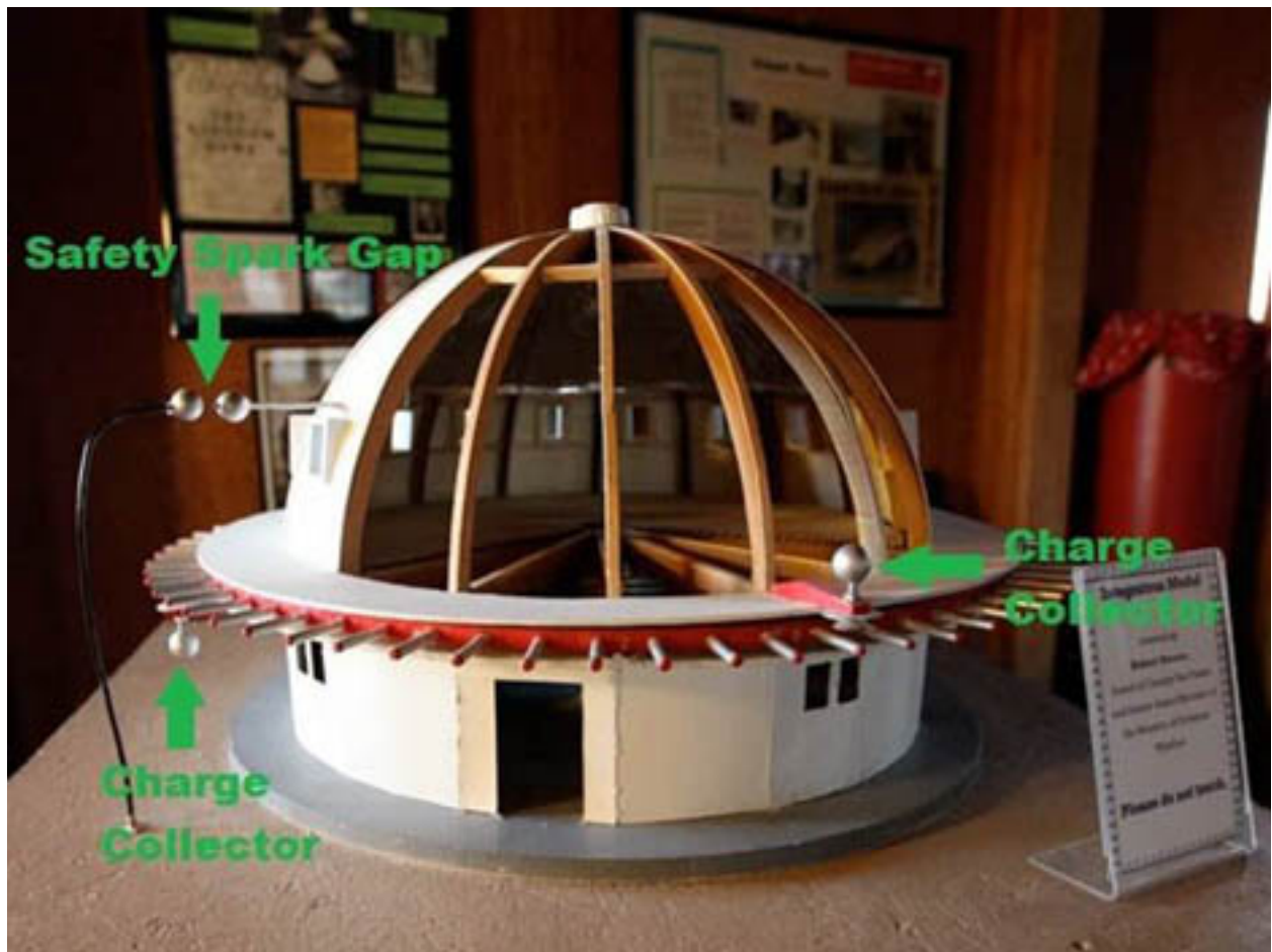
INTEGRATRON – ELECTROSTATIC TERMINAL PLACEMENT Figure 37
