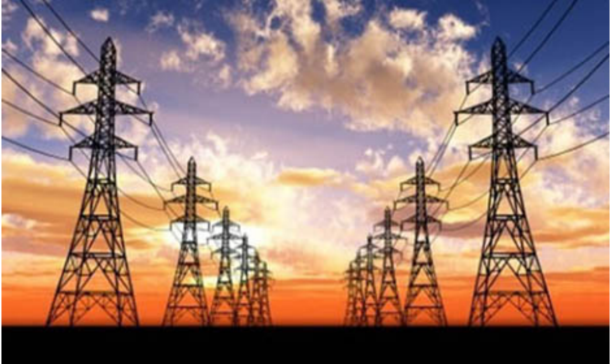
TWO DOUBLE CIRCUIT 115KV, 3-PHASE AC TRANSMISSION LINES
