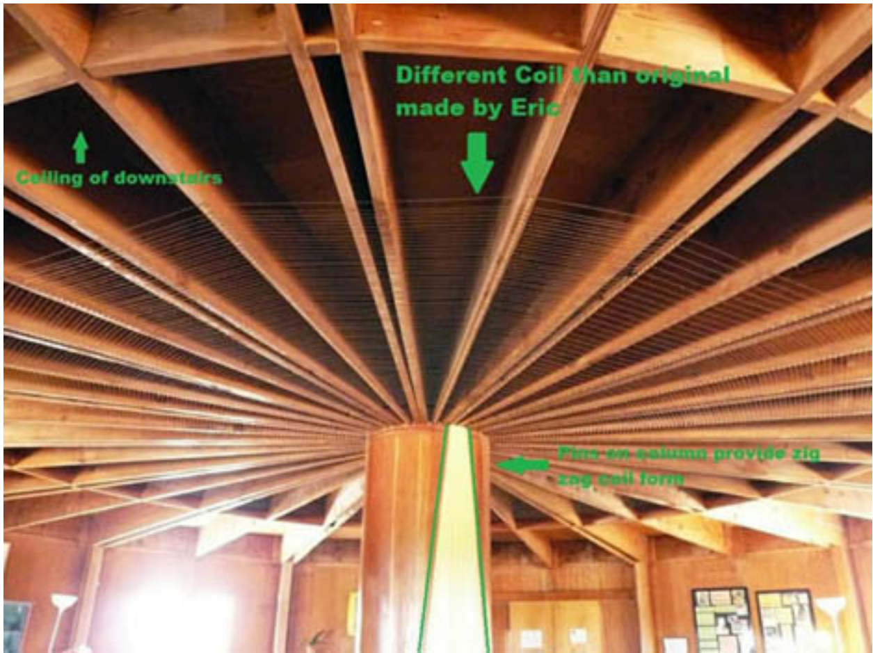
INTEGRATRON – TRANSFORMER & CENTRAL COLUMN CONDENSER (YELLOW) Figure 43
