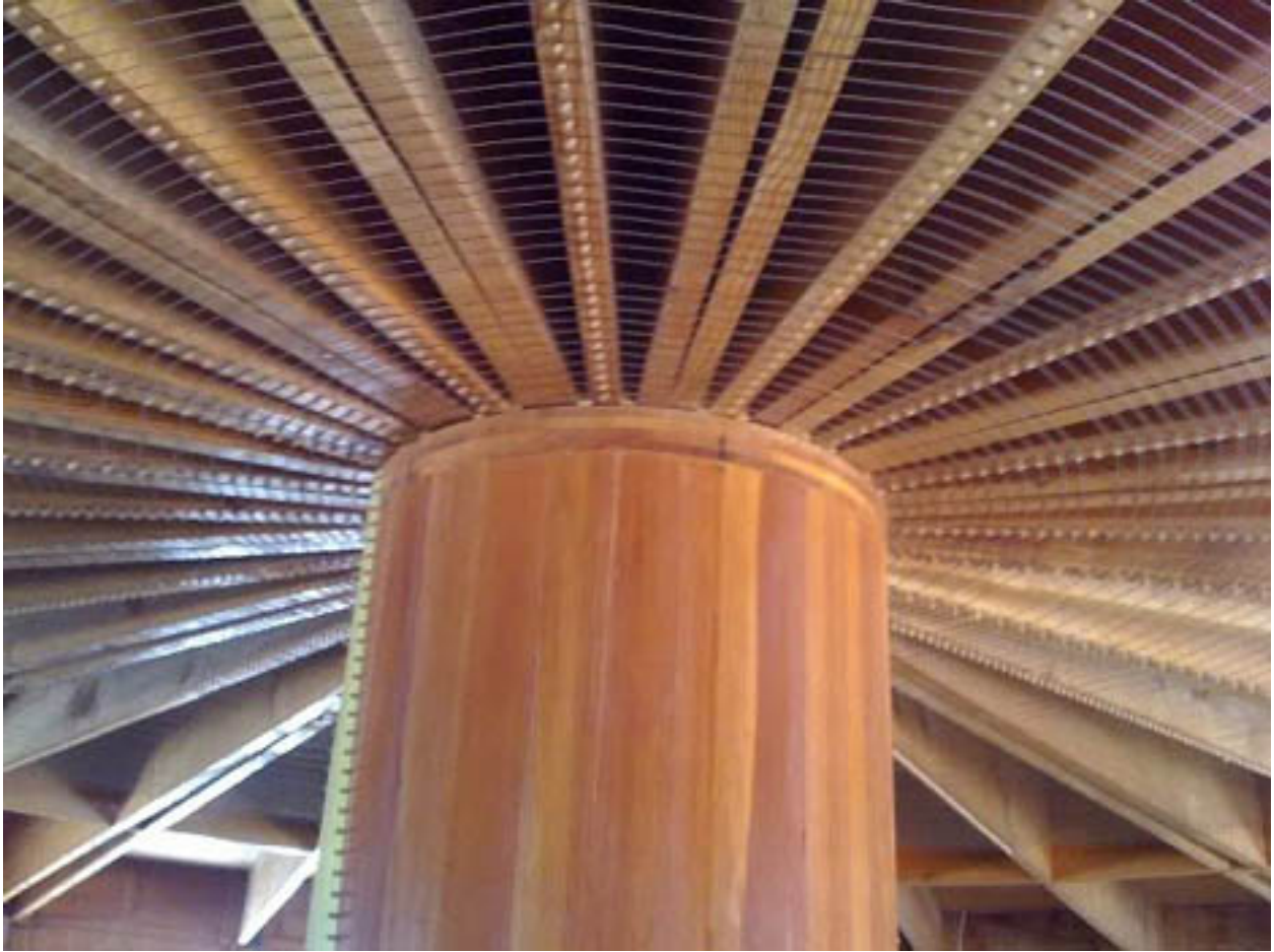
INTEGRATRON – CEILING TRANSFORMER WINDINGS & CENTRAL COLUMN
