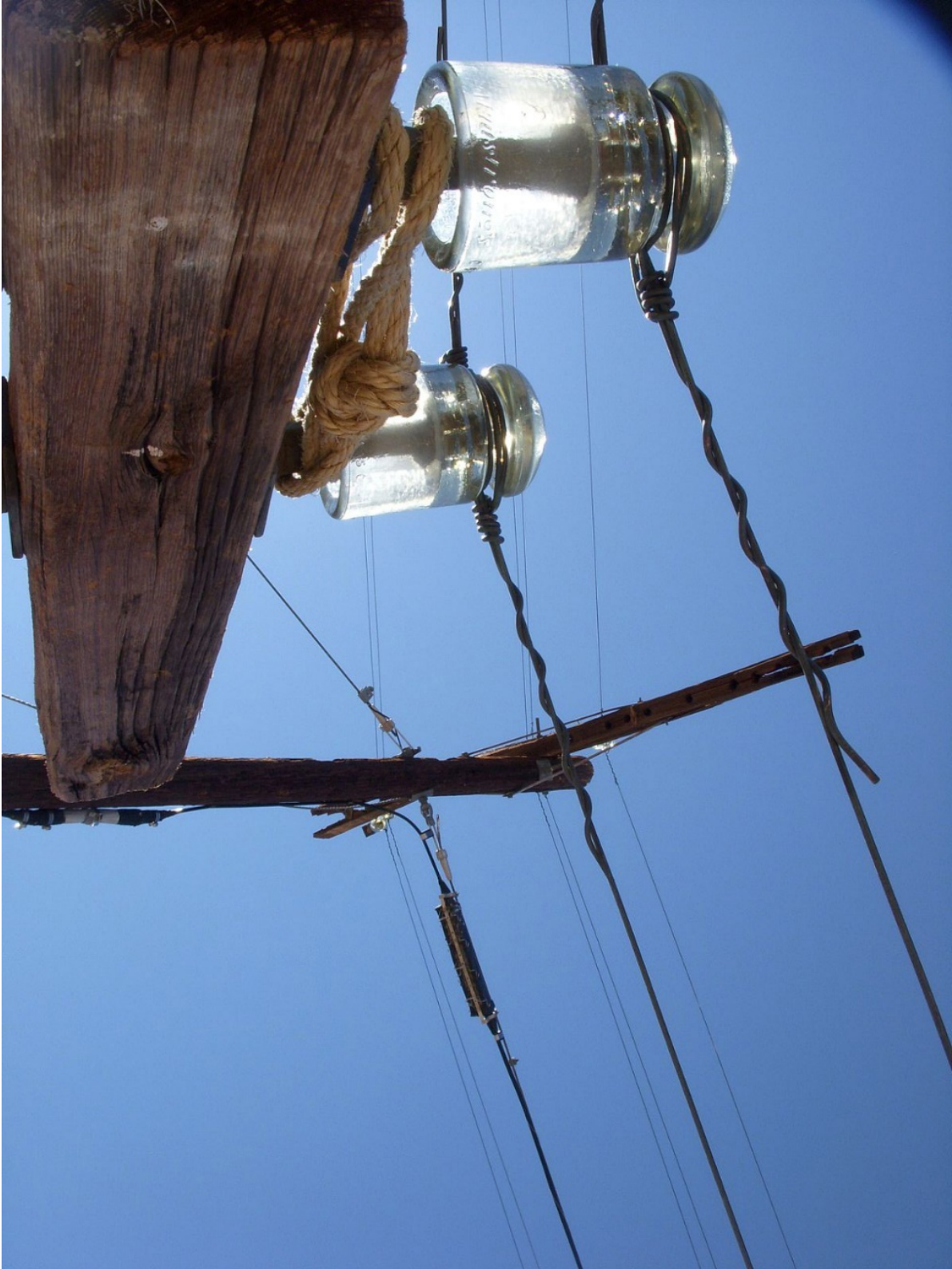
Fig. 1 - Open wire telephone transmission pair
