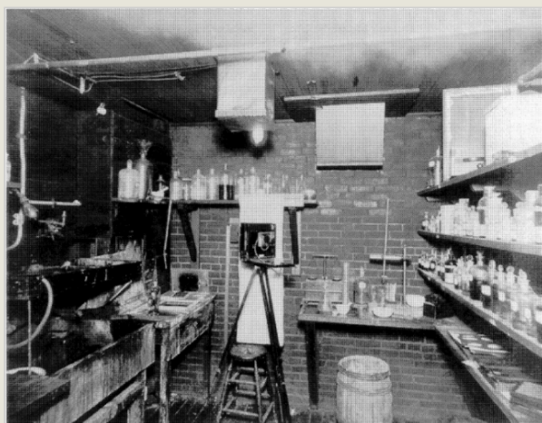
Fig. 9.3 Photographic dark room in the MIT laboratory of general physics (65 × 30 feet), with the necessary chemicals and shelving for drying the photographs (right), small balances and vials for mixing the developers and fixers, as well as a large photographic camera (center) and various containers and sinks for the developing and fixing processes. By permission of the MIT Museum, Department Photo Albums, vol. 24, no. 48.
